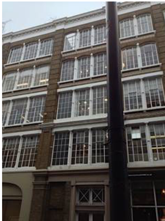
Figure 11: Bay 7 (light well)
