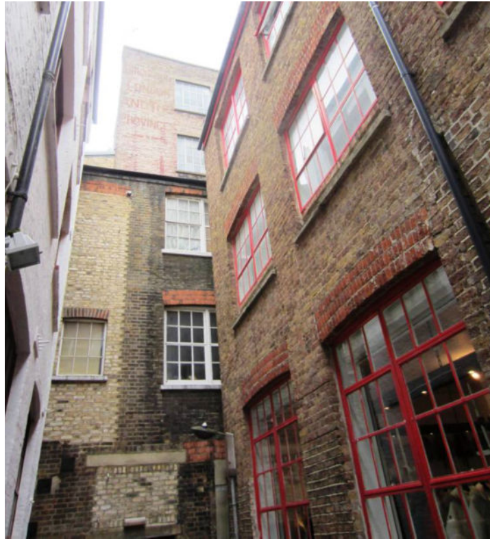
Figure 12: Rear elevation, from Elizabeth Place
